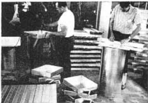
Skilled sheet metal work is performed at Owens to make many of the stainless steel units for their craft. Here galley tops are being constructed.
